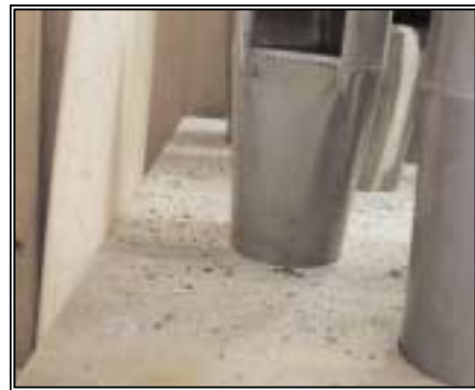
particulate dirt on the elevated Swell chest
